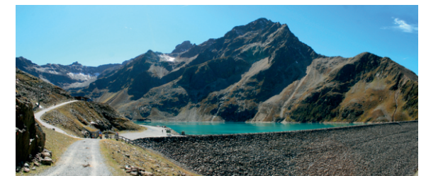
Figure E6.4: The “Finstertal” reservoir in the K uhntal/Tyrol (photo M. Weber).
